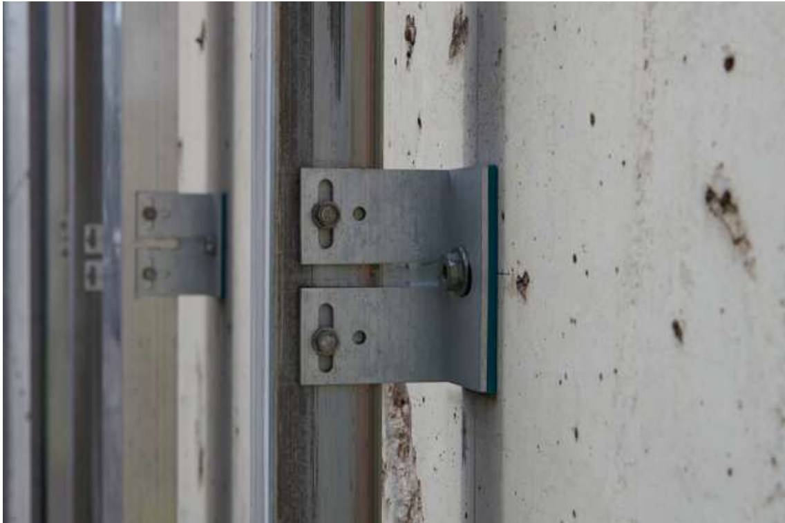
Figure 2.1.21 - Fixing the aluminium profiles to the support brackets
