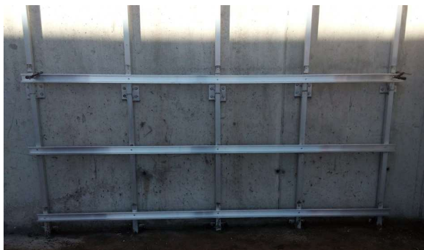
Figure 2.2.16 - View of the rail profile arranged horizontally
