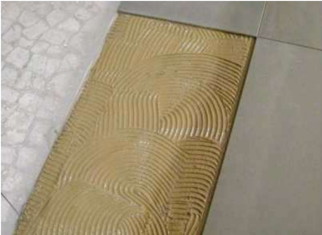
Figure 4.13 - Viroc flooring sustained on continuous support
