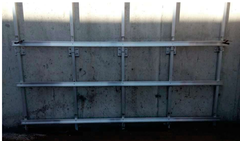
Figure 2.2.16 - View of the rail profile arranged horizontally
